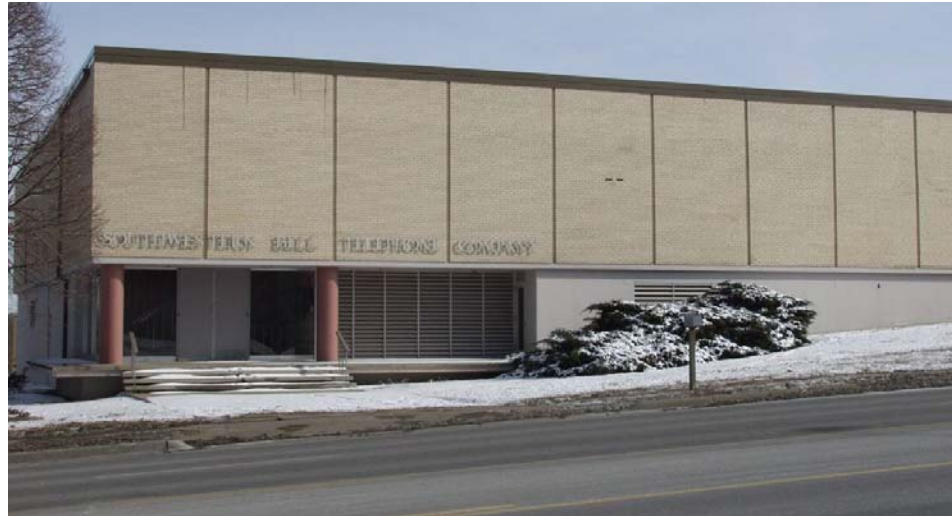
Figure 14-2: A Central Office in South Kansas City
